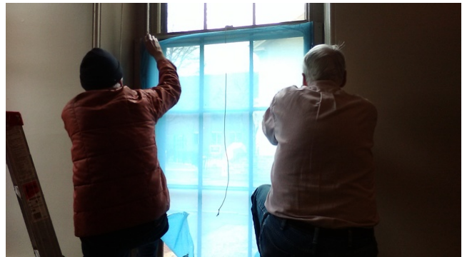
Bill and Rob fasten a panel with screws into wood strips.
