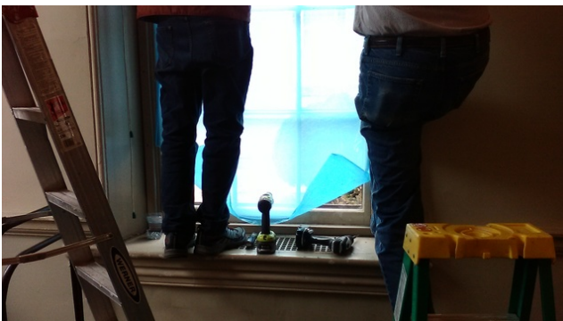
Each window had two panels, top and bottom. Before they were fastened, the blue plastic covering was removed.
